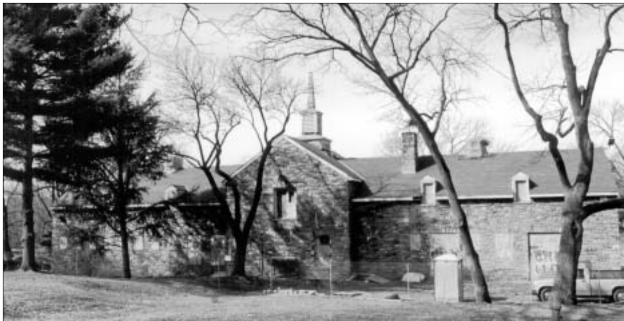
Now undergoing renovations, the historic stables at 63rd & Catherine Streets, Philadelphia, PA, a Works Progress Administration (WPA) project built in 1936 (once the home of the Fairmount Guard) will be the permanent home of the Cobbs Creek Community Environmental Education Center (CCCEEC).
