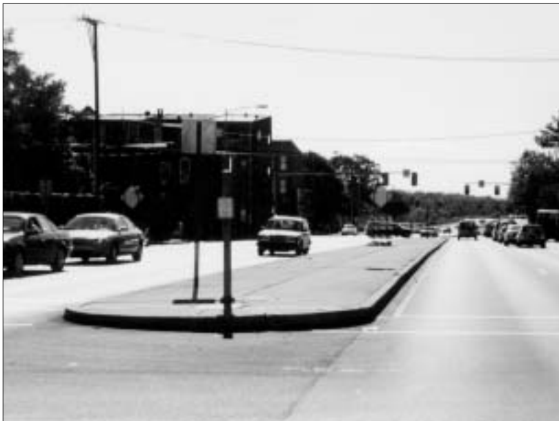
Before: Forster Street, between Second and Green Streets, 1998.
